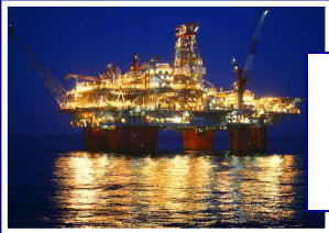
Helideck Lighting System
